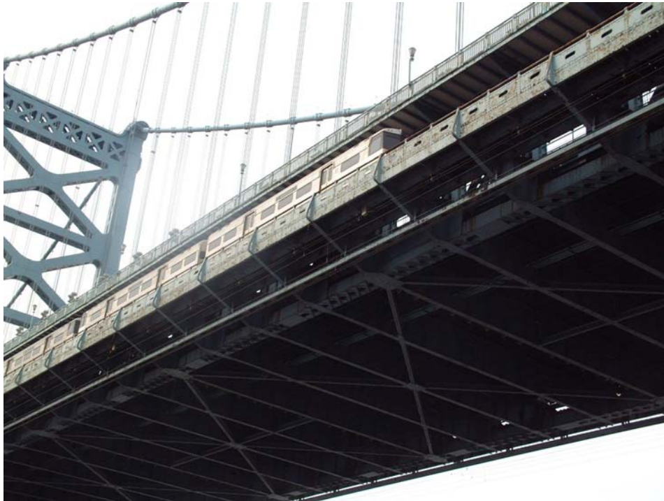
Figure 10. The Ben Franklin Bridge spans the Delaware River, with ten strain sensors periodically checking strain levels on a continuous basis at \sim 1 Hz sample rates. The presence of a passenger train creates a change in strain rate, which triggers automated data acquisition at 32 Hz sample rates by the wireless strain sensing nodes.
