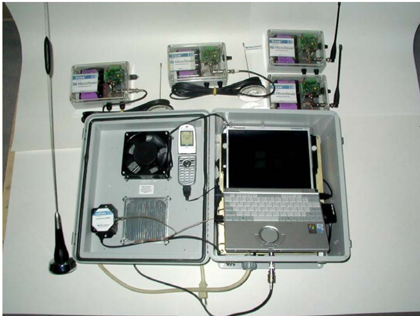
Figure 3. Wireless Sensing Nodes (4) in sealed NEMA 4X enclosures (top of photo). Base Station with Panasonic Toughbook®, cell phone, 802.11b WiFi card, and narrowband RF Transceiver as packaged within sealed, thermally controlled enclosure (at bottom of photo).
