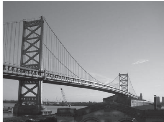
Figure 22.6.2: Ben Franklin Bridge
